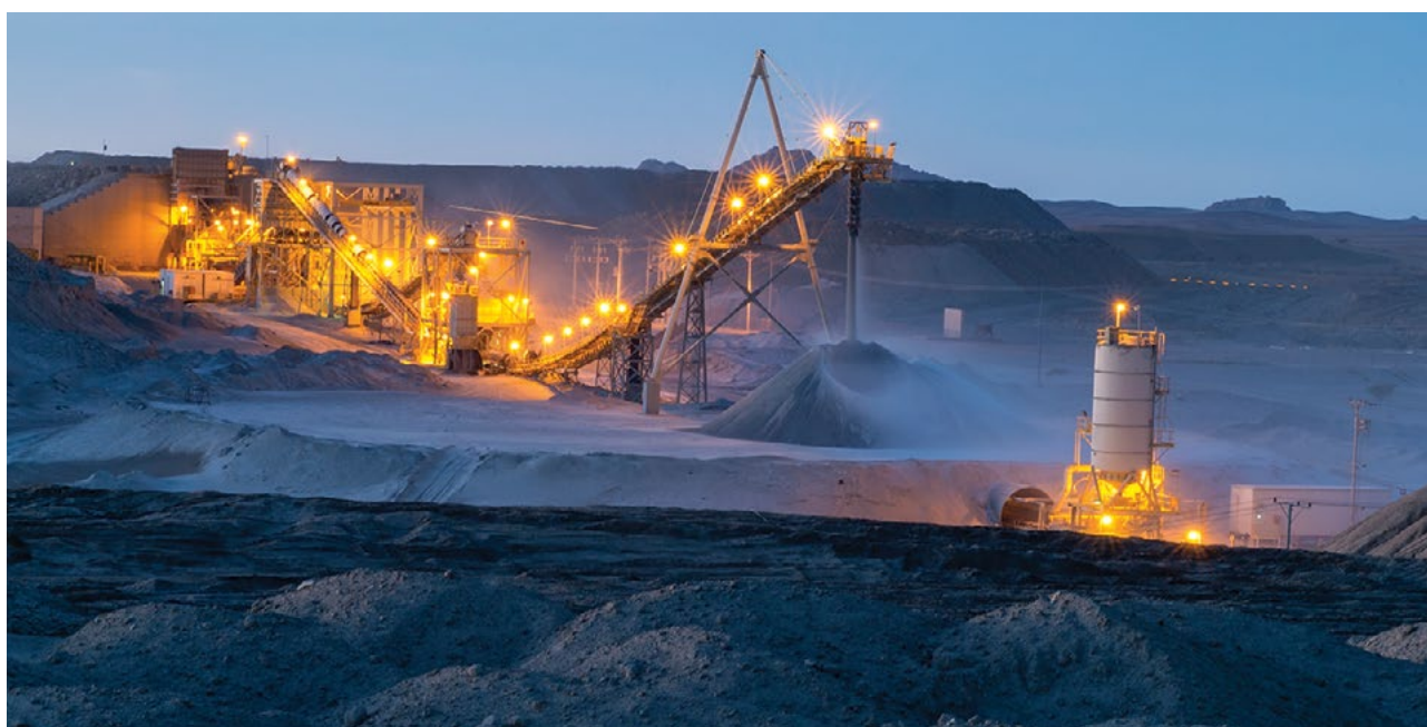
Ma'aden Gold Plant - Balgha
