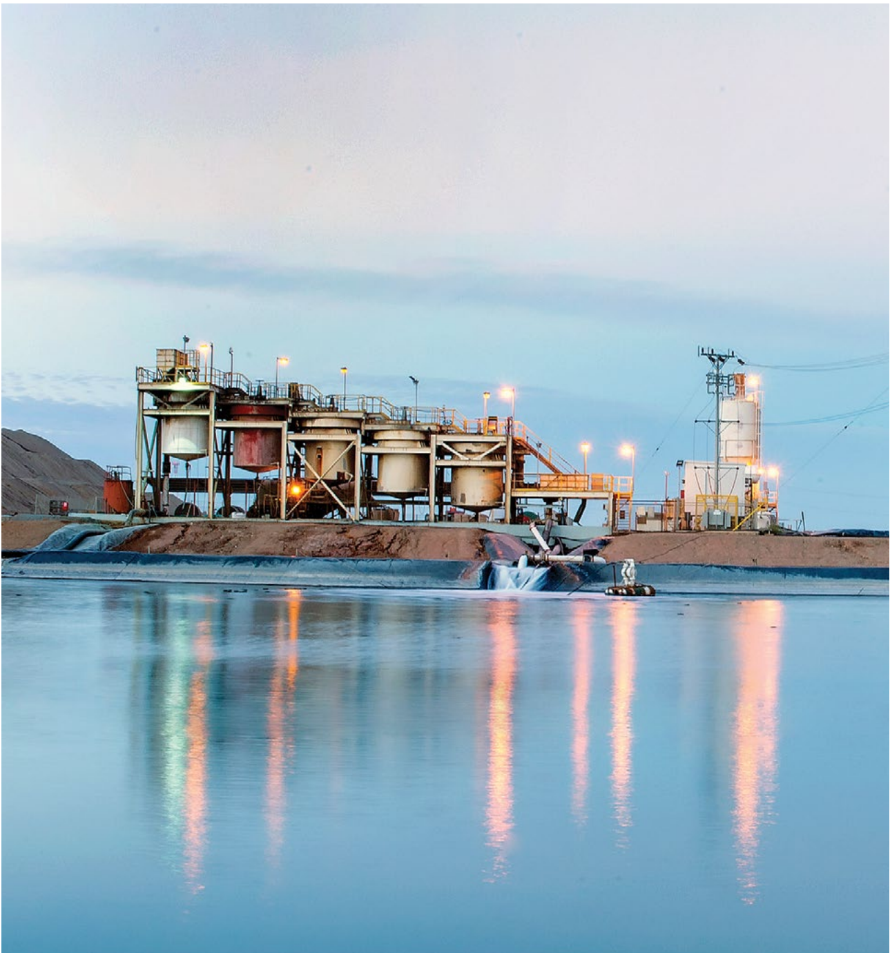
Ma'aden Gold Plant - Balgha
